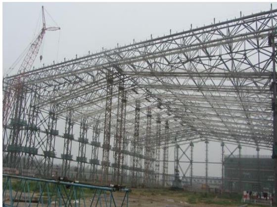
Pipe Truss installation finish
