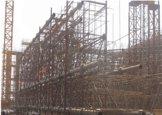
hangar door space frame assembling
