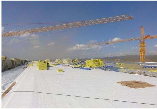
Roof Panel and insulation Installation
