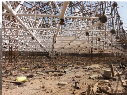
Elevation and Welding the door hangar
