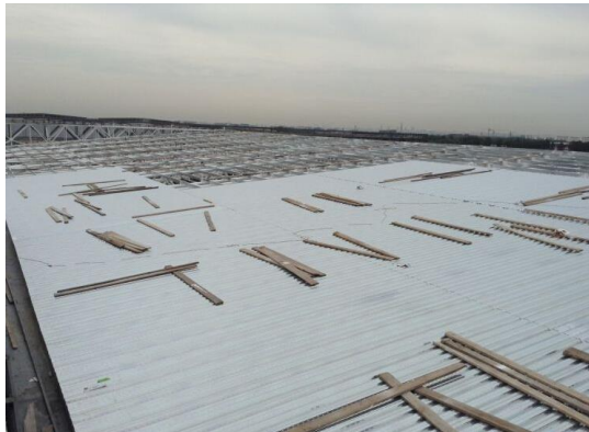
Roof profiled steel sheet installation
