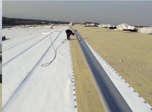
Roof TPO waterproof layer
