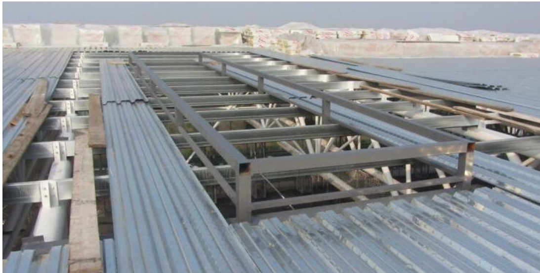
Roof Skylight Installation
