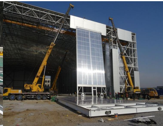
Hoisting Door installation
