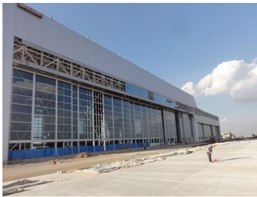
Wall glass installation
