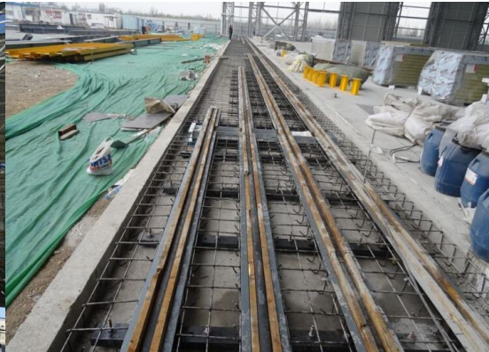
Door sliding rail installation
