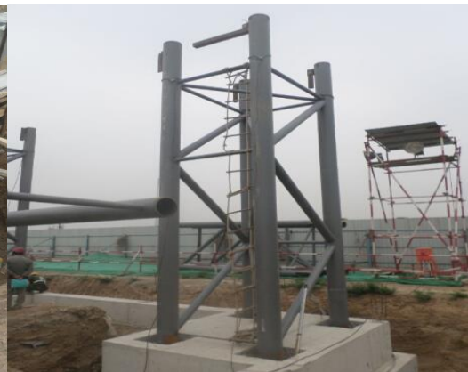
laced columns installation
