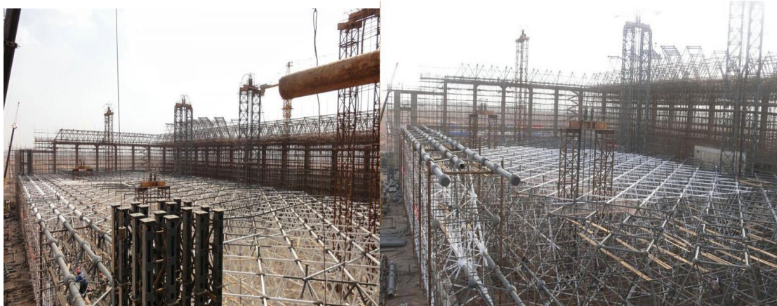
Space roof ground assembling and anti fire coating
