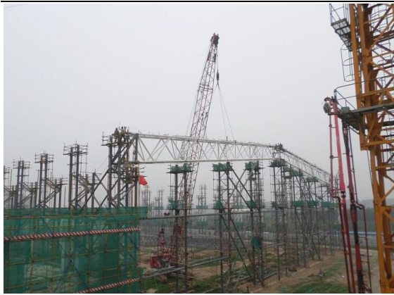
Single Truss Hoisting
