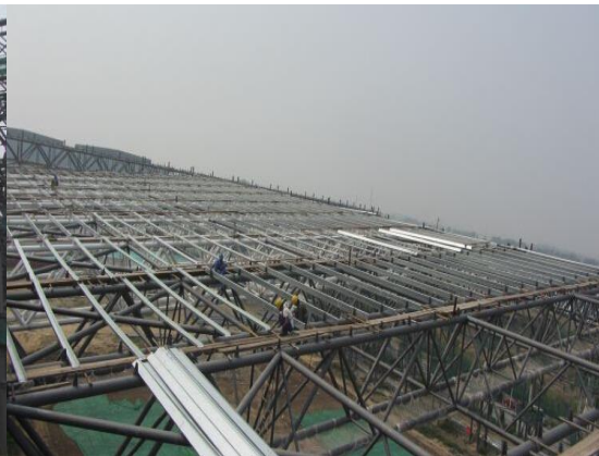
Roof Purlin Installation
