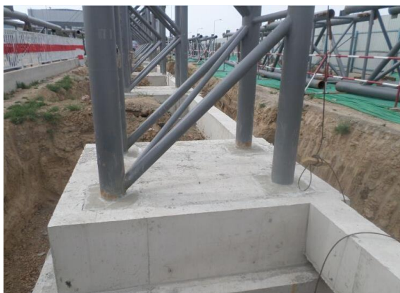
laced columns base finish
