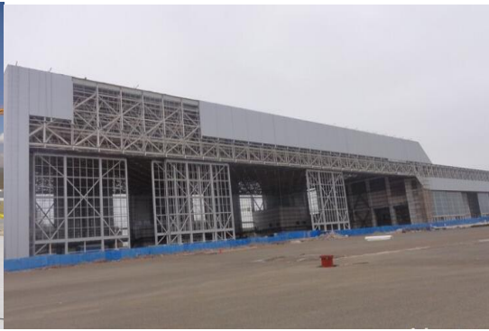
Wall panel installation
