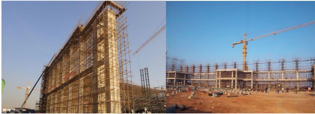
Concrete column and beam construction
