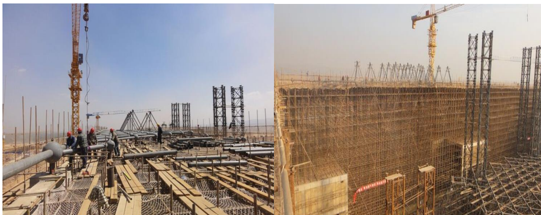
Space frame assembling aerial work
