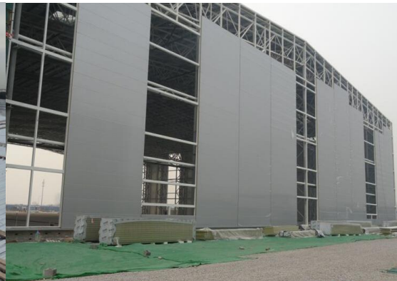
Wall Panel installation
