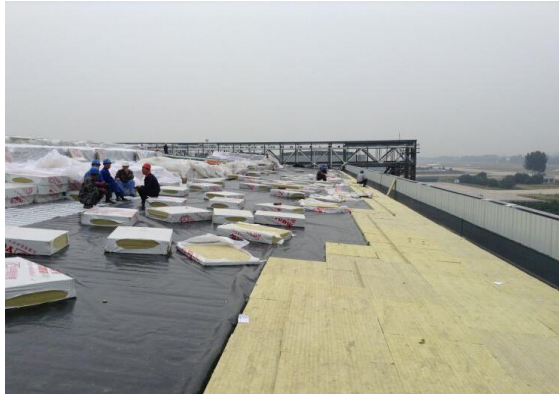
Roof Rock wool insulation
