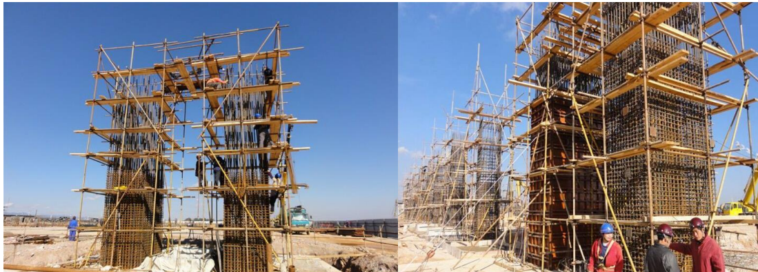
Concrete Column construction
