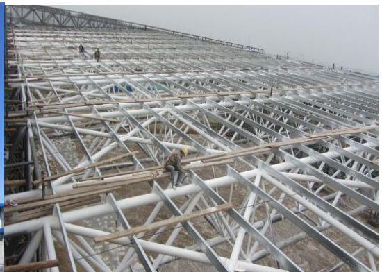
Roof Purlin/pipe truss fire-proofing coatings
