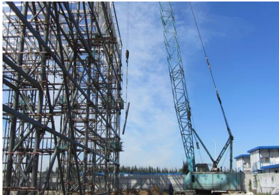
Wall Purlin Installation
