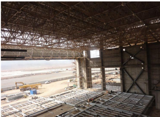
Door Assembling and Installation
