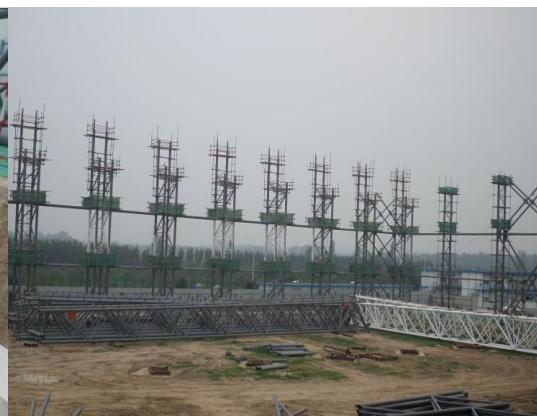
laced columns Installation finish
