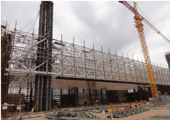
Whole set space frame elevation
